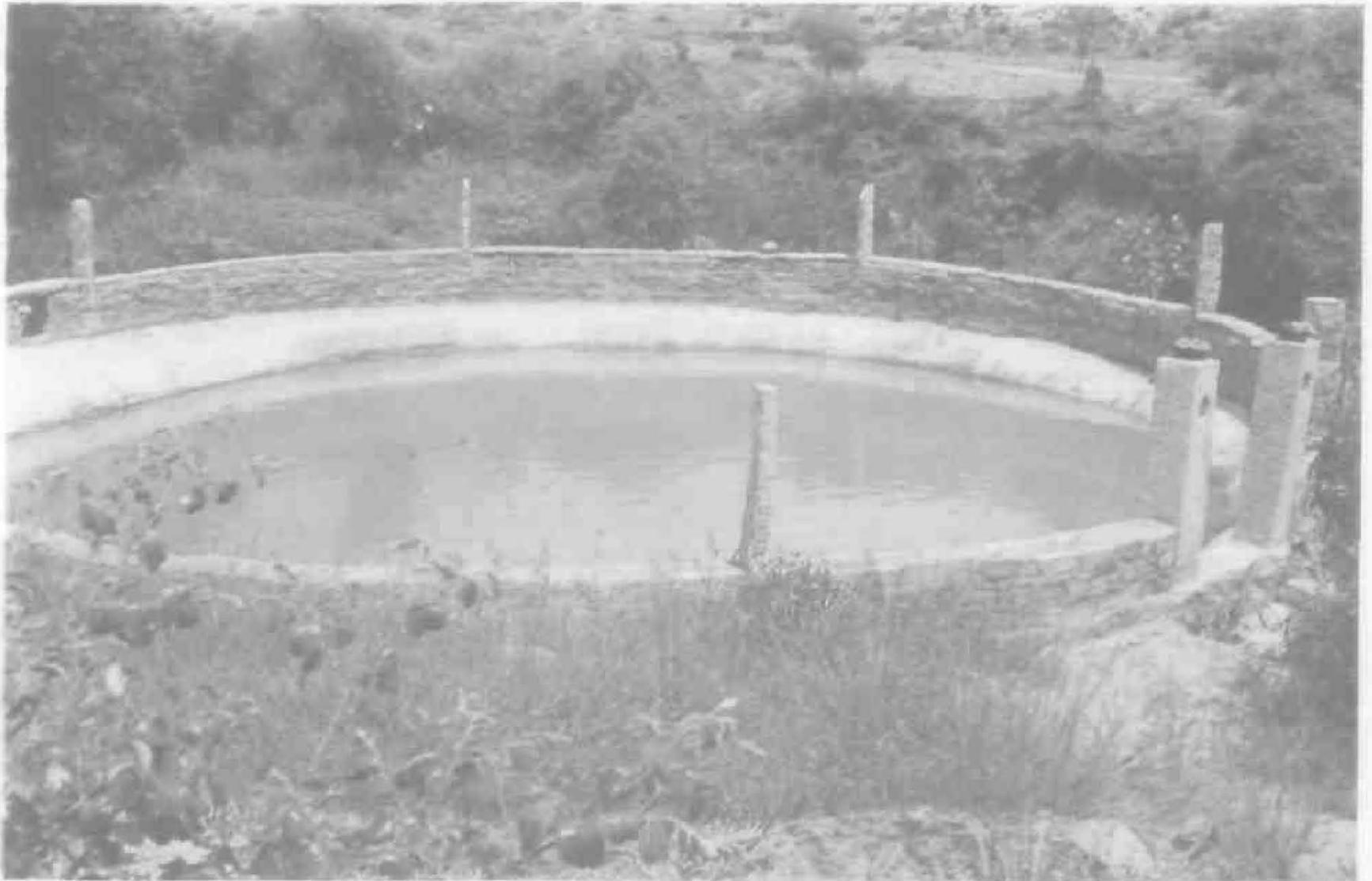
Figure 3 A farm pond of 271 m<sup>3</sup> capacity.
